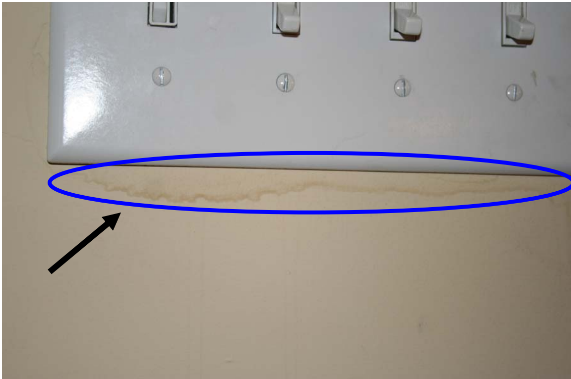
Description: Front door light switch with condensation evidence. Seal opening with gasket
