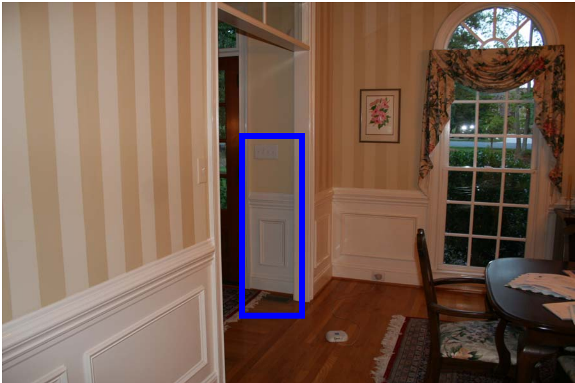
Description: Front door vent blowing on light switch with outside air leakage causing condensation
